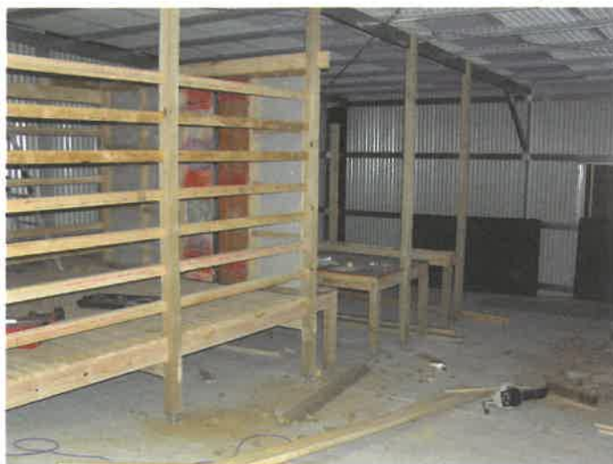
Sloping concrete floor with transverse gutter under slatted platform of holding pen; Power platform under construction
