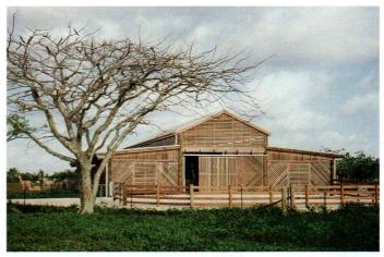
The shelter sheds, specially designed to allow maximum airflow during Niue's humid summer.
